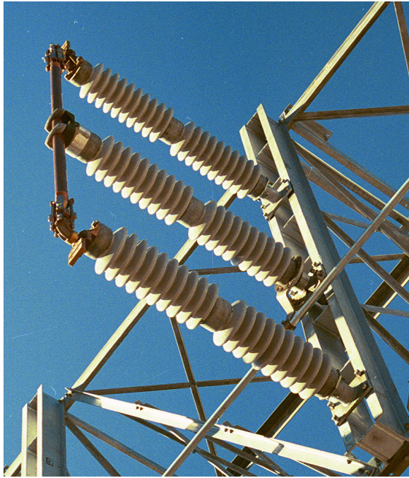
SEECO 138 kV, 2000 amp double end-break switch, catalog DV13820S
